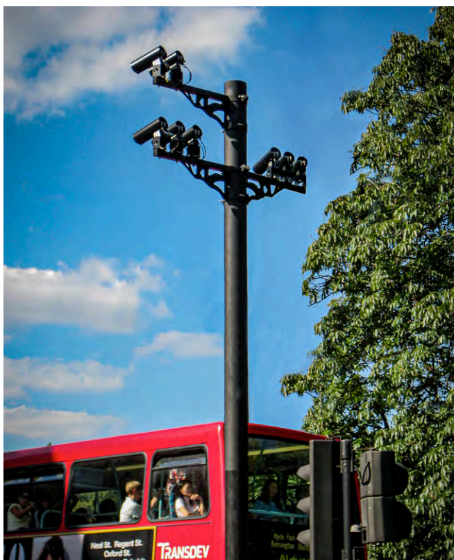
FIGURE 31: LONDON ANPR INSTALLATION
